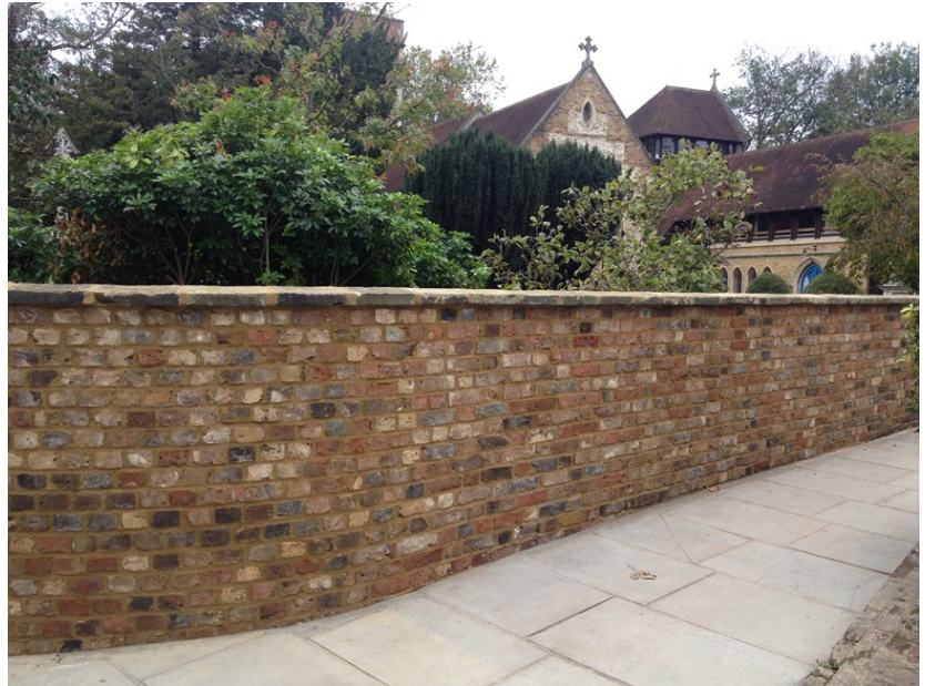
Renovated churchyard wall funded by the Friends of St Mary's
